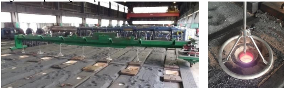
Figure 4. (a) General view of the water injection ramp in Aluchemie; (b) View of one nozzle spray injecting water in peephole 1 in Aluchemie
